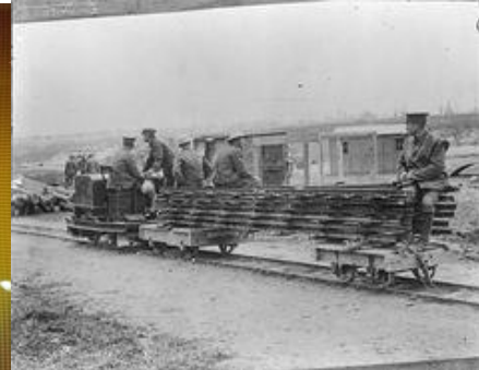
Load of track panels ready to install. Ten soldiers could easily handle them.
